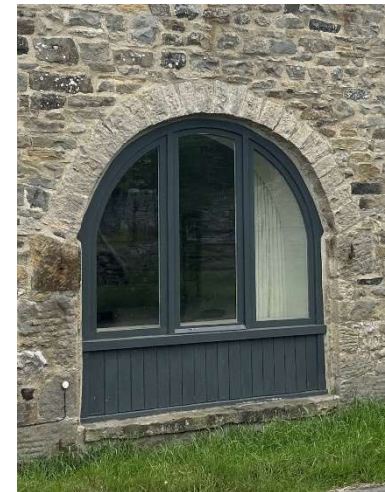
Sensitive conversion of a historic barn opening, using recessed glazing and a boarded lower panel to retain the character, scale and simplicity of the original agricultural doorway while allowing natural light into the building.
