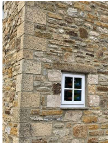
Quoins on a new extension have been textured to achieve a weathered appearance.
