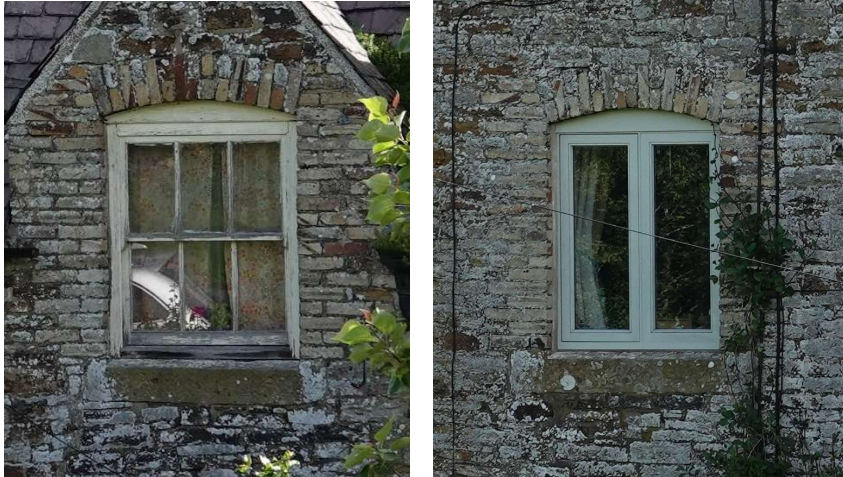
Original timber window and a replacement, illustrating how appropriate proportions and detailing can maintain the character of a historic building.
