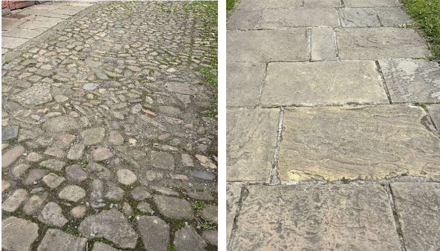
Traditional yard surfaces, including cobbles and stone flags, help define the character of the farmstead and should be retained as part of a sensitive conversion.
