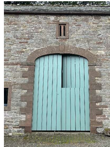
Traditional split timber doors preserve the appearance of the original barn entrance, concealing a glazed internal vestibule behind.
