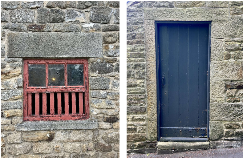
Painted timber joinery, typical of the darker colour schemes historically used on farm buildings and outbuildings.
