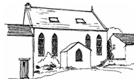
Converted chapel at Catton. The essential presence of the building is retained although the rooflights are a little conspicuous.
