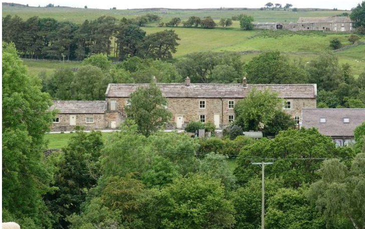
Traditional roof features including stone ridges, stone copings to gable verges and robust chimney stacks contribute to the distinctive character of buildings across the North Pennines.
