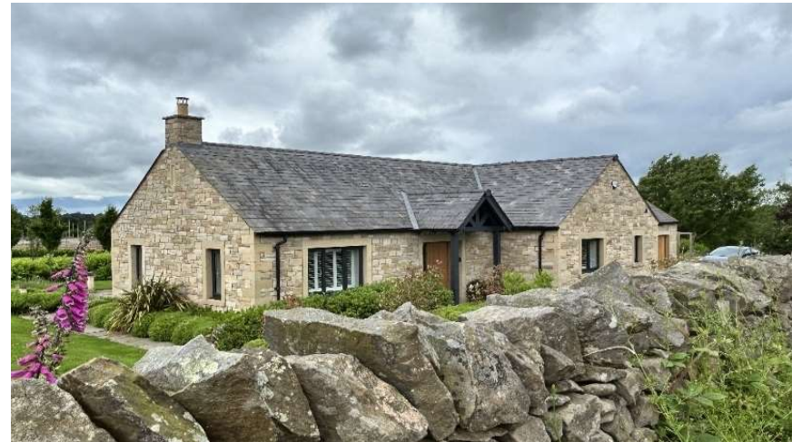
A single-storey dwelling using simple gabled forms, natural stone and slate roofs to create a low-profile development that sits comfortably within its rural setting.
