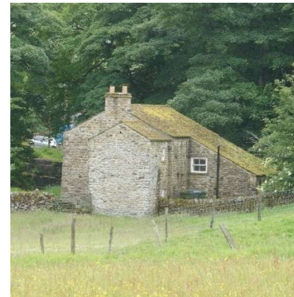
The massing of these extension remains subsidiary to the original structure
