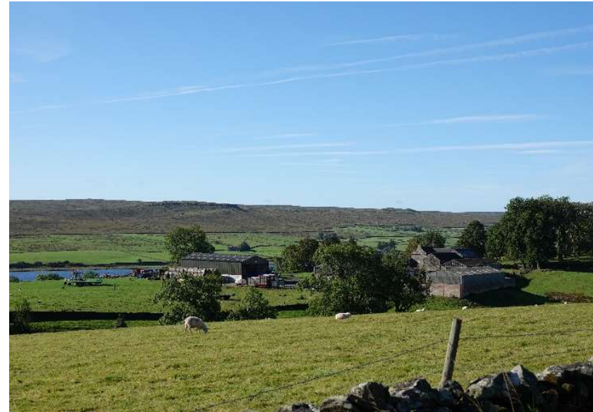
Careful siting and the use of recessive materials can help modern farm buildings integrate successfully into the landscape.
