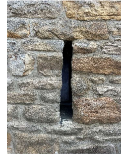
Traditional ventilation slit opening retained and fitted with a simple new insert, preserving the character of the original feature.
