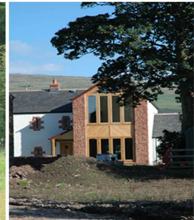
This two-storey extension, partly because of its position and manner, dominates the original house
