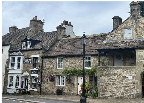
Sandstone roofing graded in diminishing courses.
