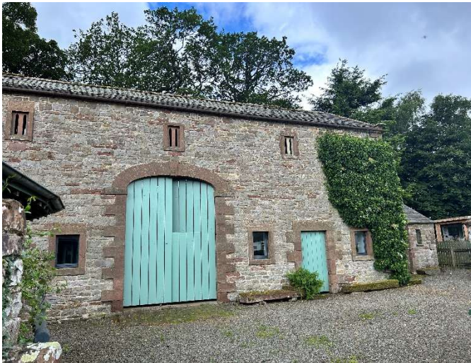
A simple conversion of a Cumbrian barn using existing openings with little loss of character.
