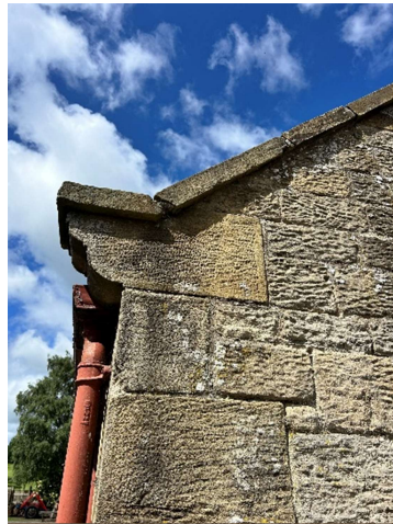
Traditional stone corbelling, coping stones and cast-iron rainwater goods retained, preserving the vernacular character and historic detailing of the building
