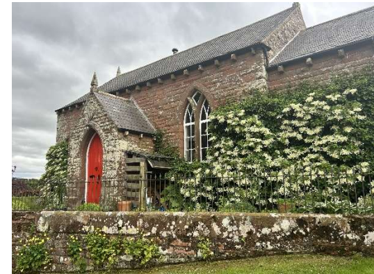
Low stone walls and simple railings can provide enclosure without creating an overly prominent boundary, particularly for historic and civic buildings.
