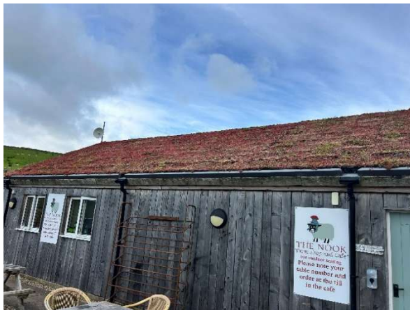
Sedum roof on a farm shop near Alston, helping to integrate the development into the landscape while delivering biodiversity and sustainable drainage benefits.
